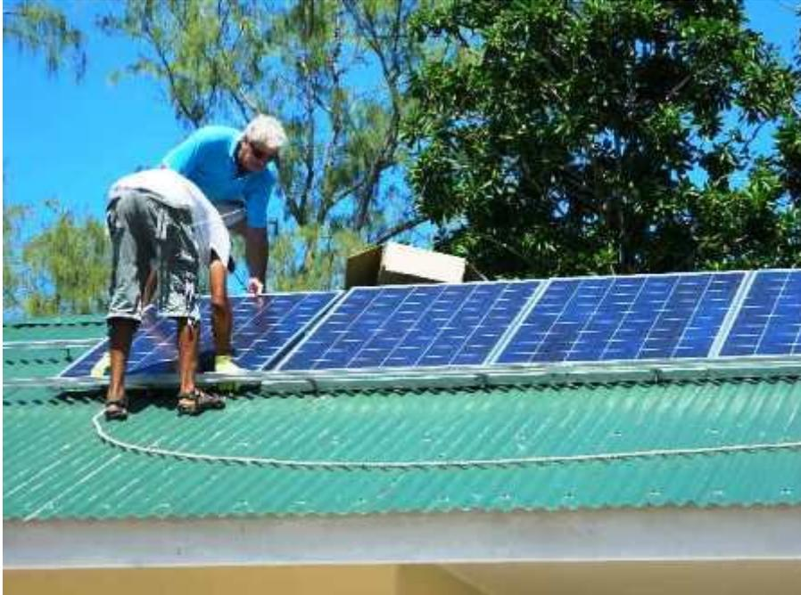
A press release from the reserve – whose details we hope to publish on Saturday – says the island is now functioning on solar power from a newly installed renewable energy system comprising a series of panels, a 5 kilowatt inverter and 20 batteries.
